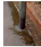
Moss on hard surfaces
