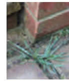
Weeds in paving
