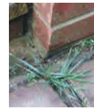
Weeds in paving
