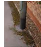
Moss on hard surfaces
